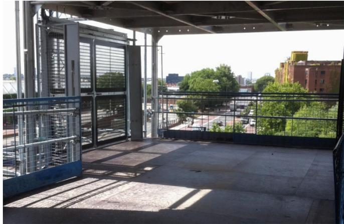
As only the common tower, and not the hoists, are tied directly into the building, it means external cladding can be applied to the whole building during construction with the exception of the 4.5 metre access openings at each level. As a result there are far fewer panels to replace at the end of the project, which dramatically speeds up de-rigging.
