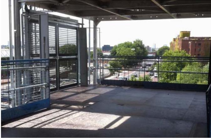
during construction with the exception of the 4.5 metre access openings at each level. As a result there are far fewer panels to replace at the end of the project, which dramatically speeds up de-rigging.
