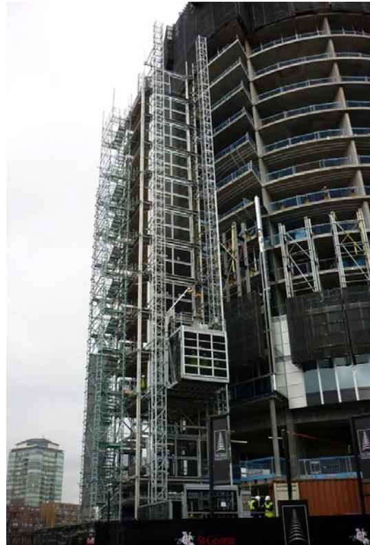
Manufactured from aluminium alloy to minimise weight, and fully stress tested by RIFI, the CAS common tower has a mere 5 x 5 metre footprint yet is capable of running multiple hoists simultaneously. This allows all material and personnel hoists to be concentrated in one area, which streamlines loading efficiency at ground level. With all hoists operating simultaneously it minimises waiting times for men and materials, especially at peak times.
