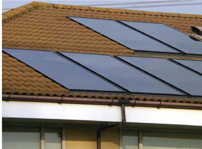
roofline remains flush and watertight. As well as being more aesthetically pleasing it means there is no additional load on the roof, so they can be fitted without any modification to the roof structure.
