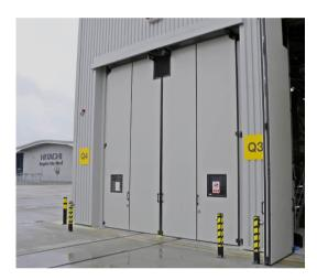
At the front of the building, Jewers installed four of its latest generation Swift-SEW bi-folding doors, specifically designed for the rail industry. Each comprises four highly insulated, single
