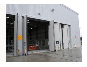
piece composite panels, with two leaves folding to each side on the outside of the building. Leaves are operated by a newly developed high power centrally mounted drive unit which incorporates inverter control for smooth start and stop and takes less than 10 seconds to open the door fully. Operator safety is ensured with full height pressure sensitive safety edges and photocell beams to create a safe zone around
