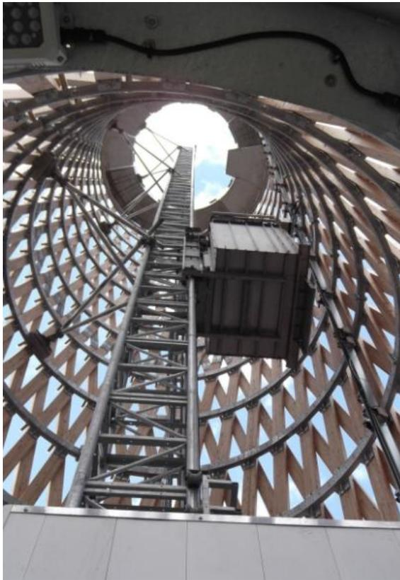
The stunning self-supporting hyperboloid sculpture is made from a lattice of glulam (glued laminated) PEFC certified Siberian Larch laths supported by a series of steel rings. The structure is illuminated at night by over 600 low energy LED lights which can be programmed for both intensity and colour to achieve a range of visual effects.
