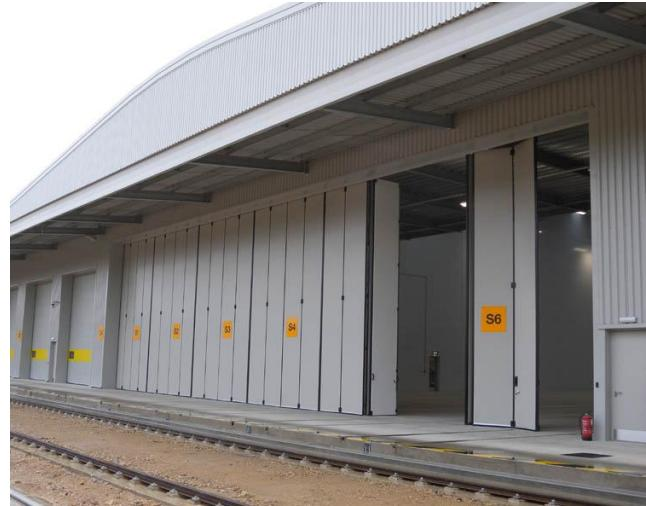
All Phoenix doors are manufactured from single piece, fully insulated panels with CFC-free polyurethane core to optimise thermal efficiency and reduce noise pollution by up to 25dB. The panels are seamlessly fitted with multi-wall rubber seals to all edges to reduce water, air and dust ingress and all hardware is maintenance-free.
