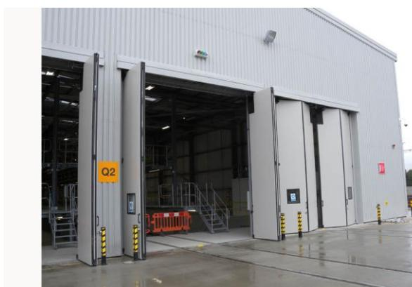
the door. Each door closes around an OLE and when open leaves are locked in position
